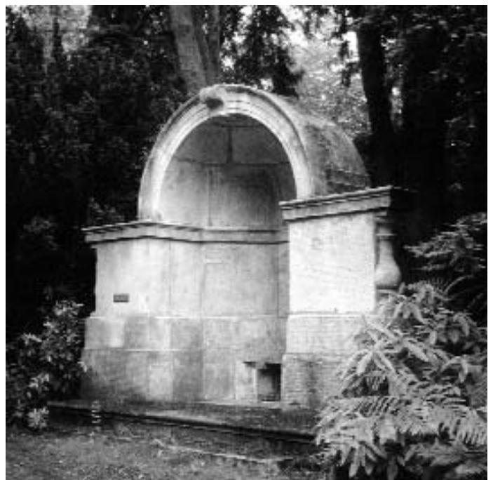
'This alcove was purchased at the demolition of Old London Bridge and brought to Hedsor Wharf and thence by horse-waggons to Dropmore. It was first laid on the grass at the back of the pinetum and in 1839 erected on its present site by Lady Grenville.' Text from the plaque visible on the left side of the structure.
