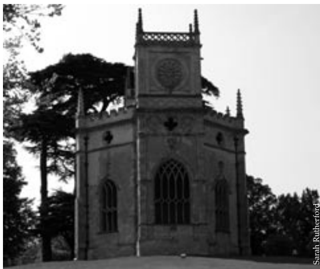
Hartwell's now redundant church on its mound near the house
